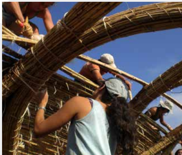
Cane construction techniques developed by the spanish collective Canya Viva.
